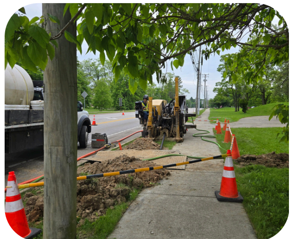
Contractor Performing Directional Drilling
