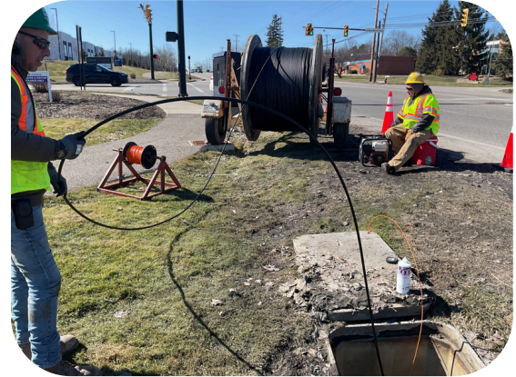
Reel of Fiber Being Installed
