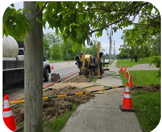
Contractor Performing Directional Drilling
