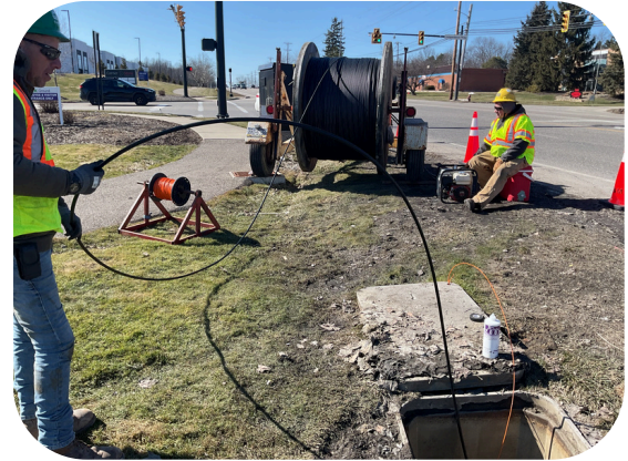
Reel of Fiber Being Installed
