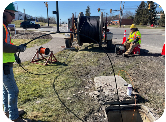
Reel of Fiber Being Installed
