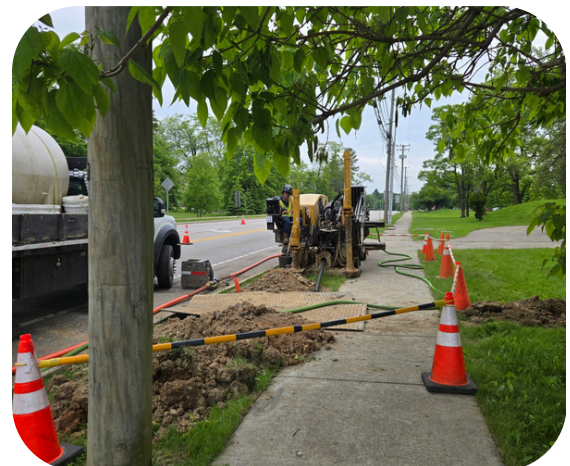
Contractor Performing Directional Drilling
