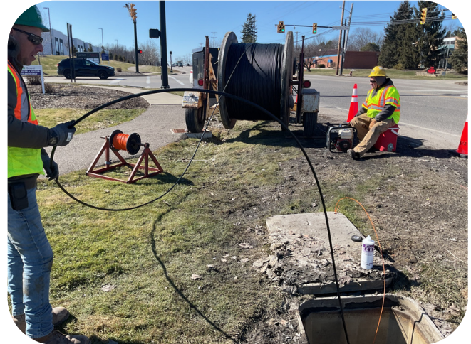
Reel of Fiber Being Installed
