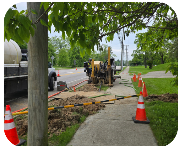
Contractor Performing Directional Drilling
