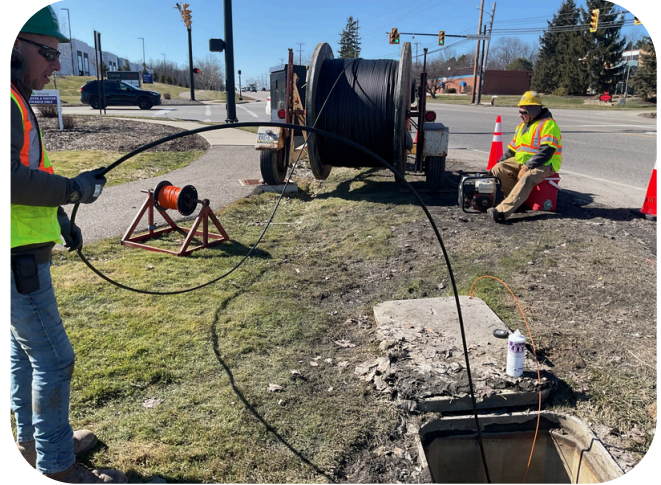
Reel of Fiber Being Installed
