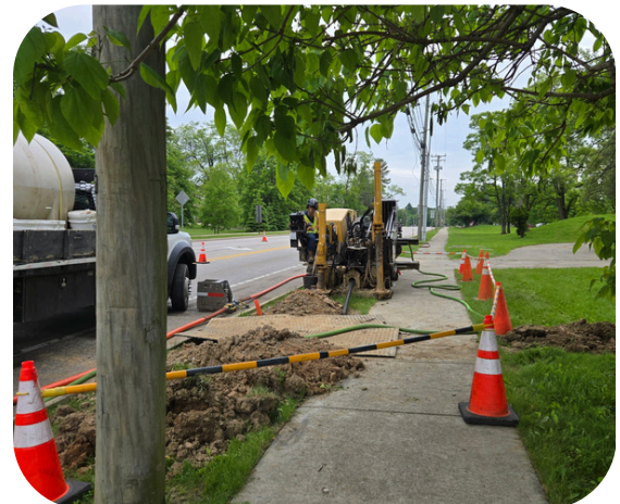
Contractor Performing Directional Drilling
