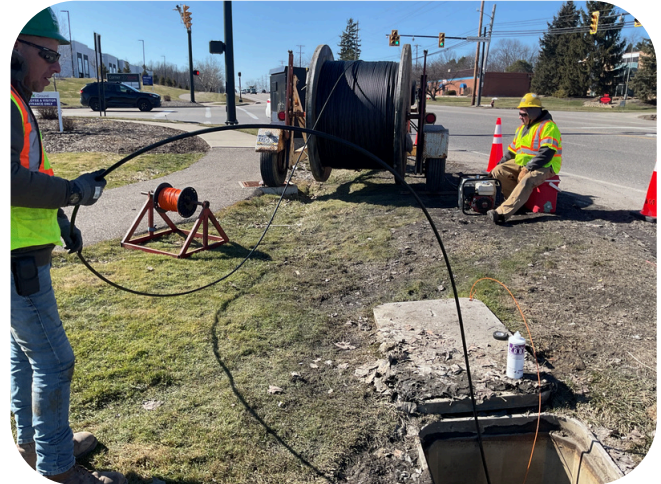
Reel of Fiber Being Installed
