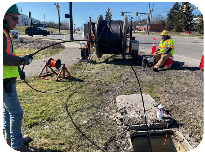
Reel of Fiber Being Installed
