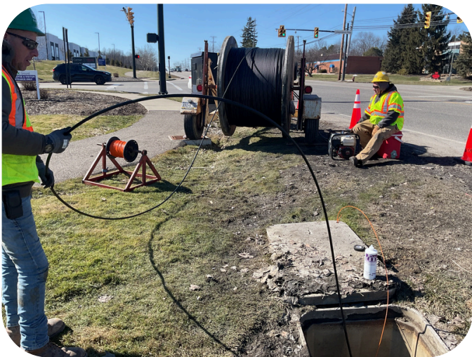
Reel of Fiber Being Installed
