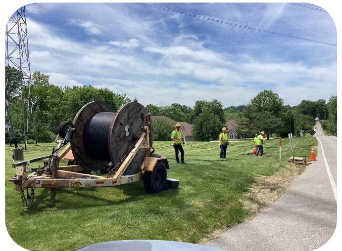
Reel of Fiber Being Installed
