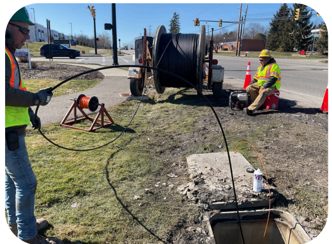
Reel of Fiber Being Installed
