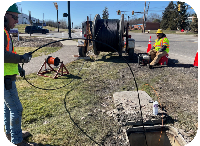
Reel of Fiber Being Installed
