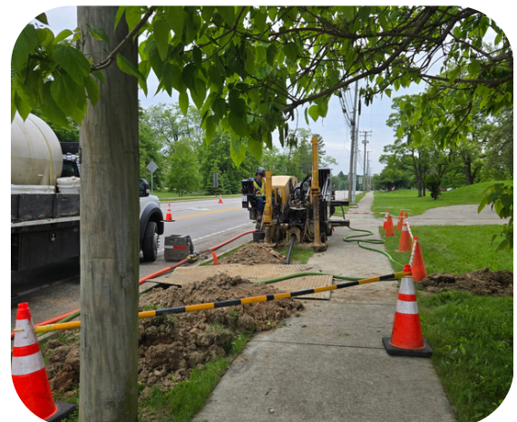
Contractor Performing Directional Drilling
