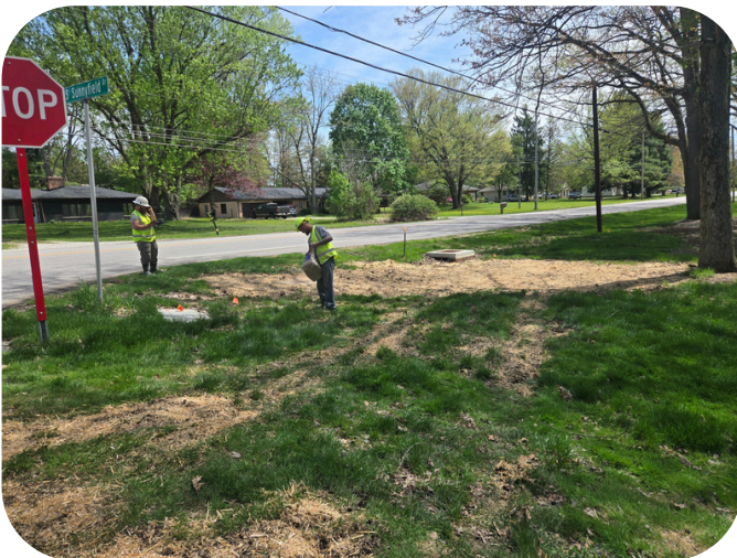
Restoration in Progress
