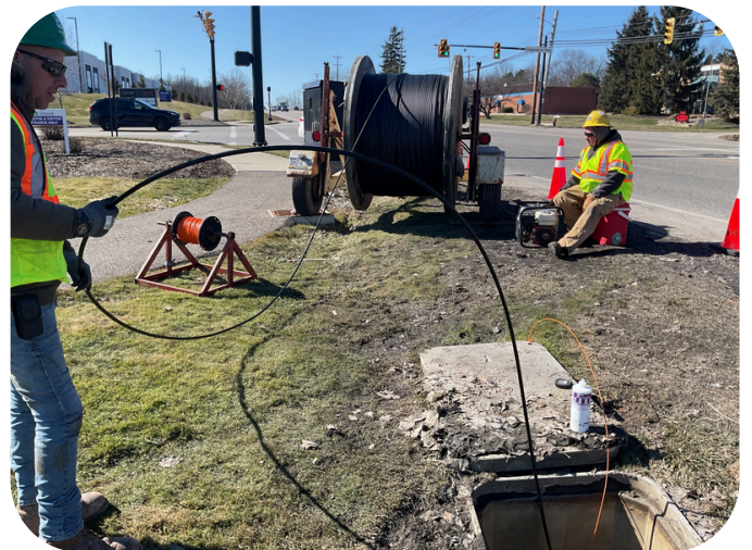
Reel of Fiber Being Installed
