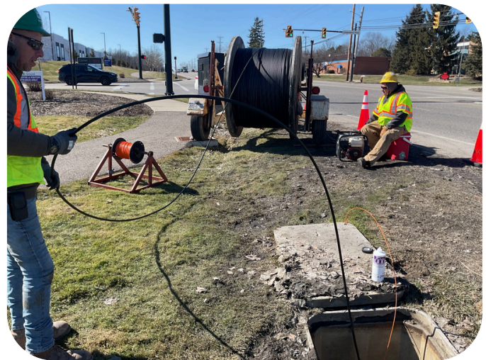
Reel of Fiber Being Installed
