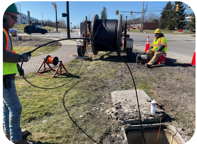
Reel of Fiber Being Installed
