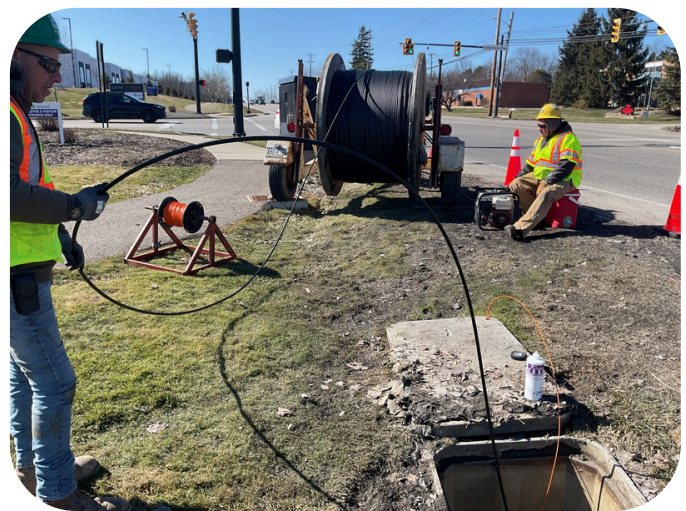
Reel of Fiber Being Installed
