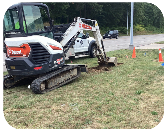
Staging Setup for a Pull Box
