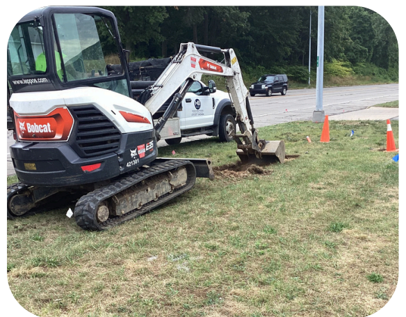
Staging Setup for a Pull Box
