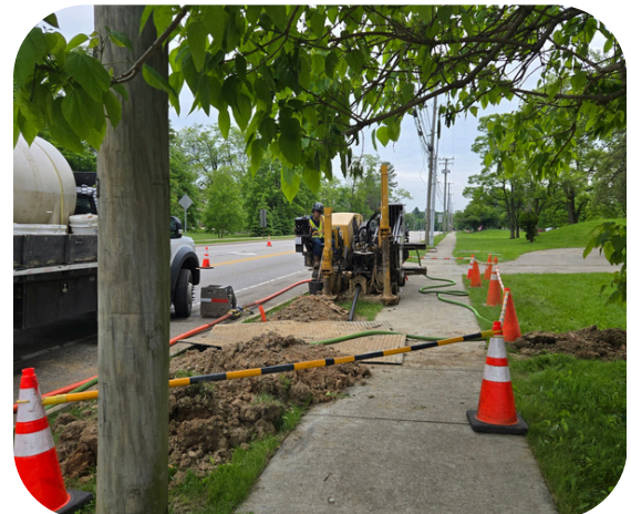
Contractor Performing Directional Drilling
