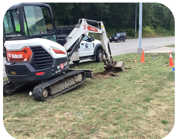
Staging Setup for a Pull Box
