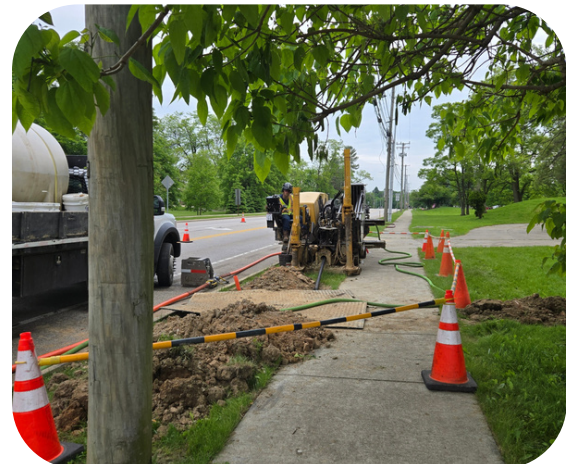
Contractor Performing Directional Drilling
