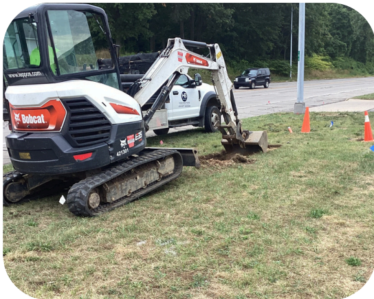
Staging Setup for a Pull Box
