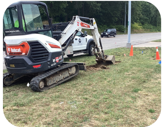
Staging Setup for a Pull Box
