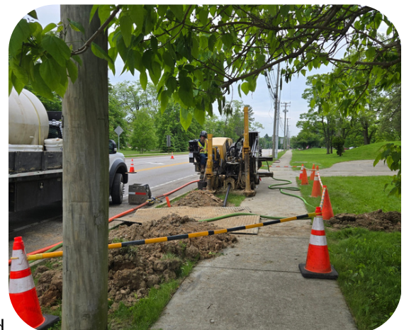
Contractor Performing Directional Drilling
