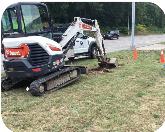
Staging Setup for a Pull Box
