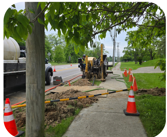
Contractor Performing Directional Drilling
