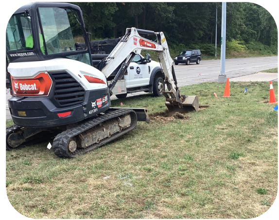
Staging Setup for a Pull Box
