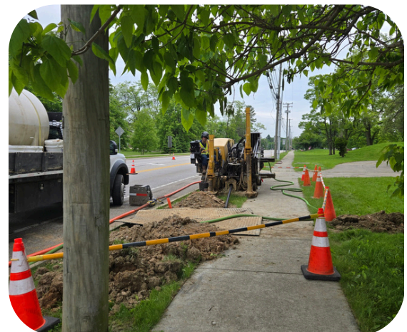
Contractor Performing Directional Drilling
