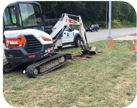
Staging Setup for a Pull Box
