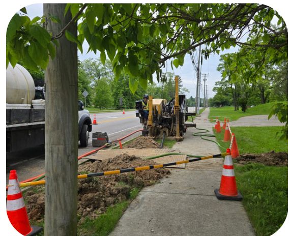
Contractor Performing Directional Drilling
