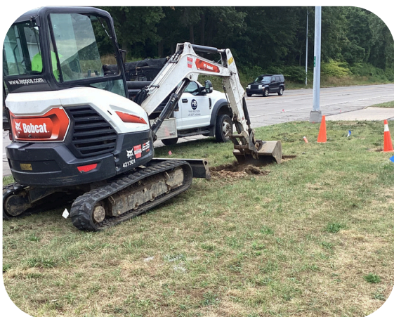
Staging Setup for a Pull Box
