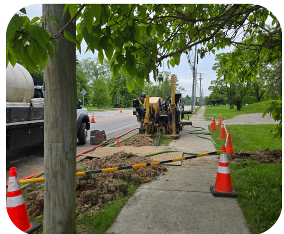
Contractor Performing Directional Drilling
