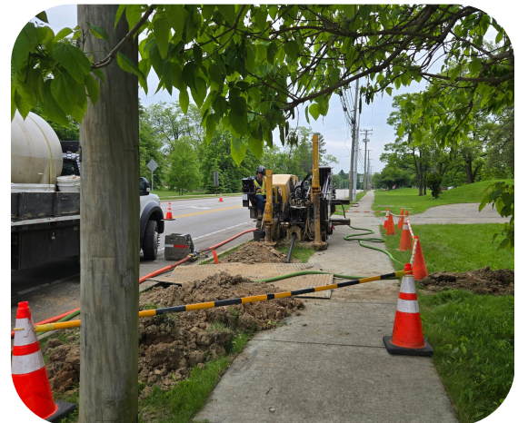
Contractor Performing Directional Drilling
