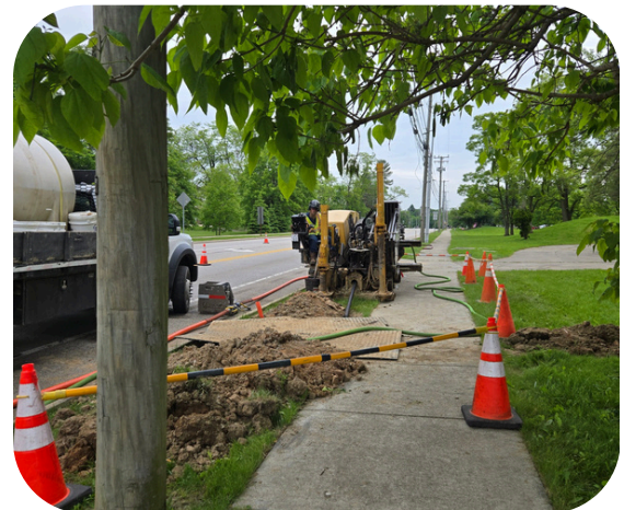
Contractor Performing Directional Drilling
