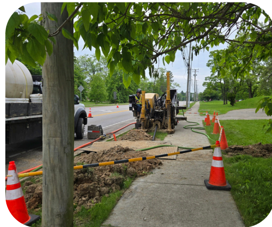
Contractor Performing Directional Drilling
