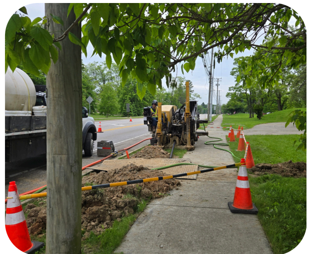
Contractor Performing Directional Drilling
