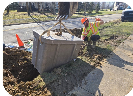
Pull Box Installation
