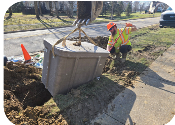
Pull Box Installation
