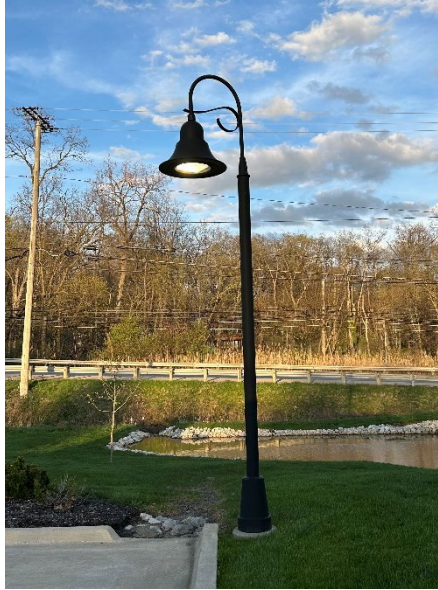
Figure 604-B – Cut-off light fixture example
