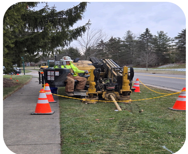
Contractor Performing Directional Drilling
