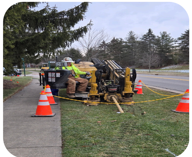
Contractor Performing Directional Drilling
