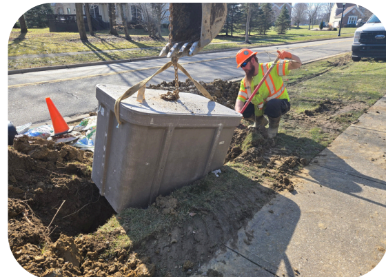
Pull Box Installation
