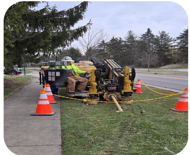
Contractor Performing Directional Drilling
