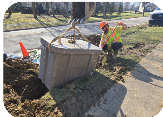
Pull Box Installation
