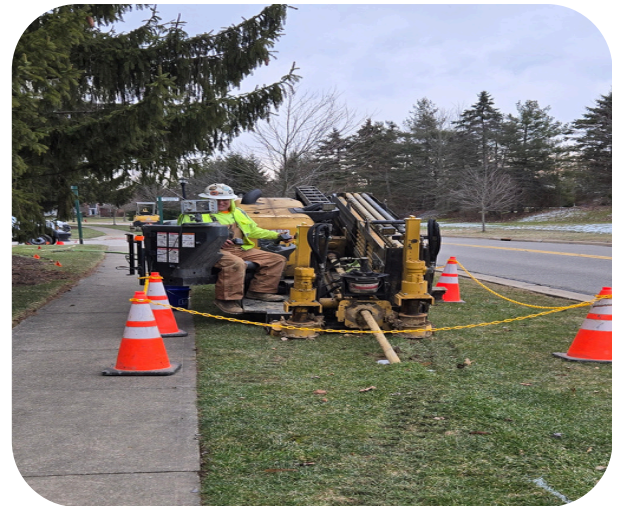
Contractor Performing Directional Drilling
