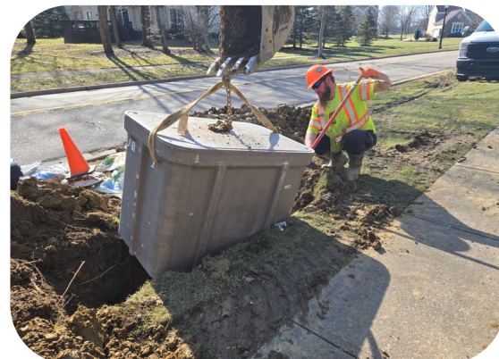
Pull Box Installation
