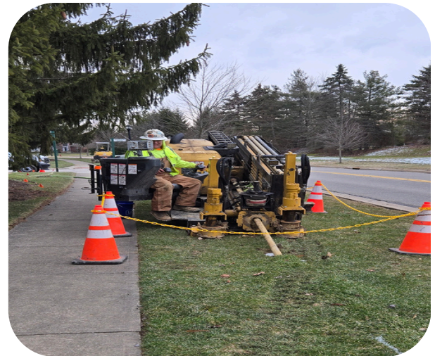
Contractor Performing Directional Drilling
