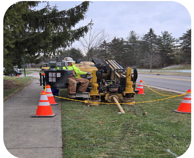
Contractor Performing Directional Drilling
