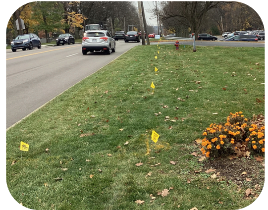
Yellow Utility Locator Flags Please do not remove these flags
