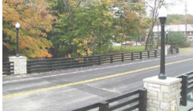
Figure 3: The Wye Road bridge in Bath Township was designed to allow views through the side railings—drivers, cyclists and pedestrians can “see the water.”
